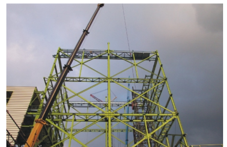
Westfalenhütte galvanizing plant of Number 8 hot-dip coating line, Dortmund
